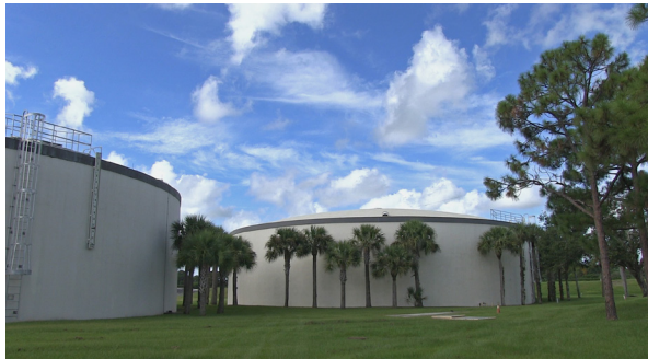
St. Lucie West Services District uses SCADA to control 53 lift stations and five different processes.
