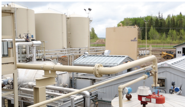
The old SCADA system at Enerchem's Slave Lake facility was not very manageable.
