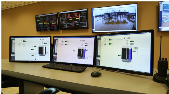
The central control room featuring eight monitors, with two 4K monitors, and two virtual annunciators
